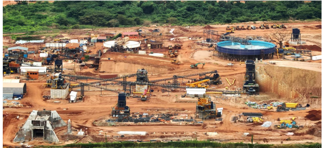
Construction for MRM's second processing plant, as seen in 10 March 2025
