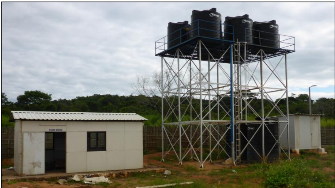
Figure 8-6: Namanhumbir Camp Potable Water Storage Tanks
