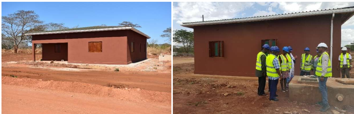
Image: All houses have now been completed by the contractor
