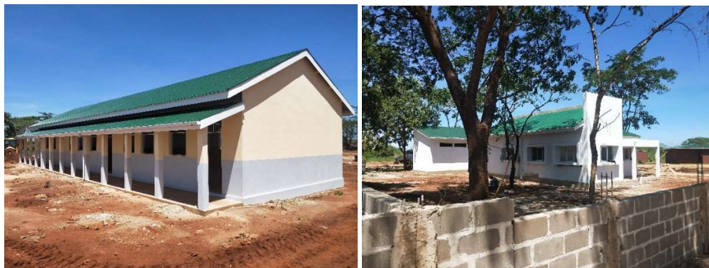
Image: Public buildings nearing completion
